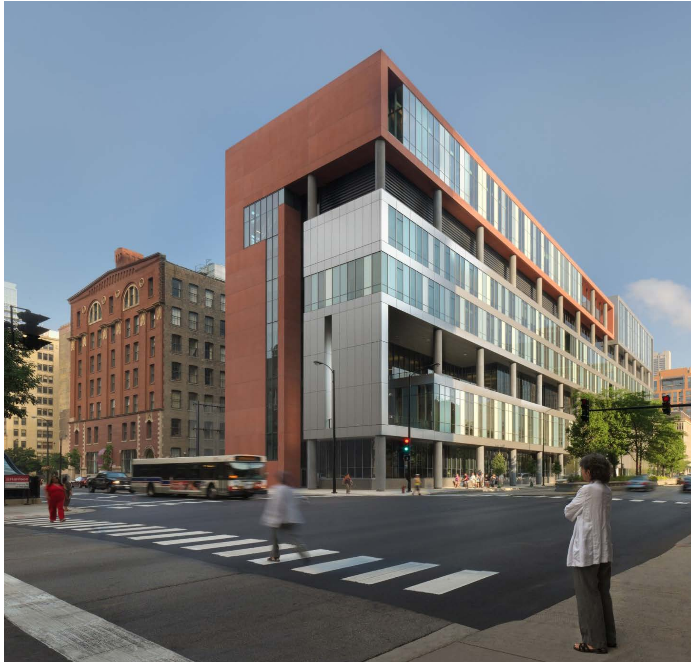
LINCOLN HIGH SCHOOL MODERNIZATION DAG 8 | MARCH 14, 2019
