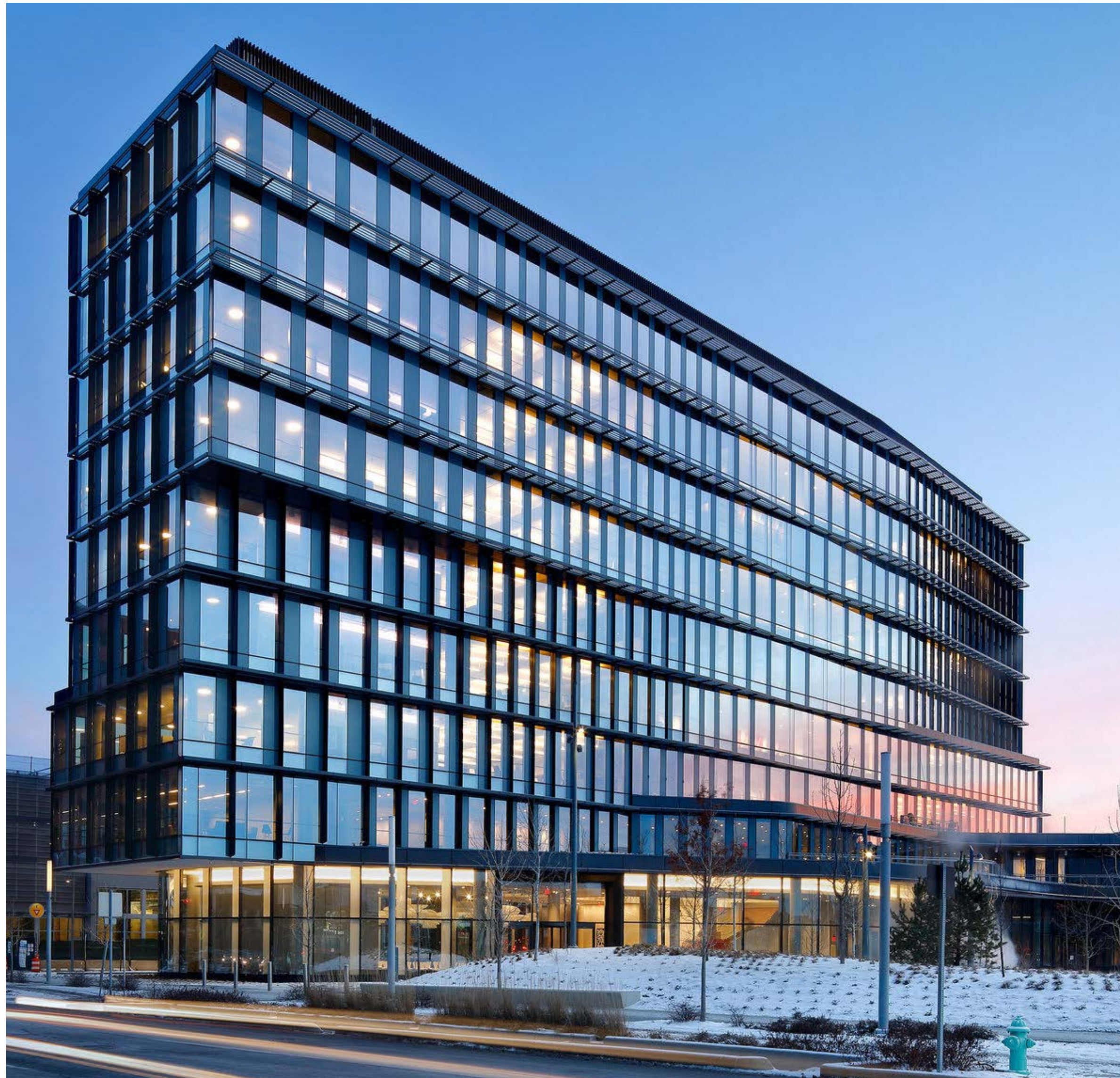
LINCOLN HIGH SCHOOL MODERNIZATION DAG 8 | MARCH 14, 2019
