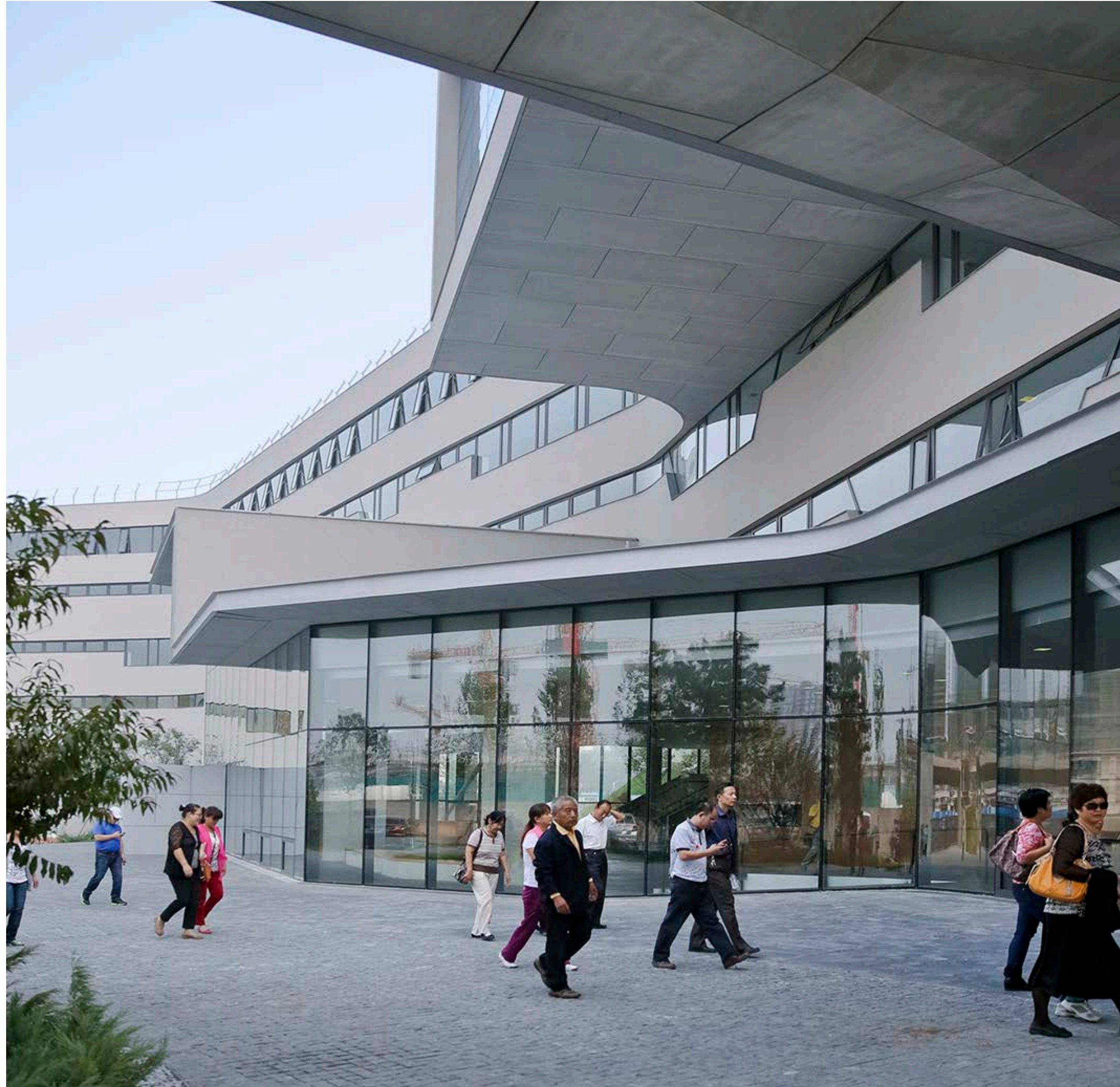
LINCOLN HIGH SCHOOL MODERNIZATION DAG 8 | MARCH 14, 2019
