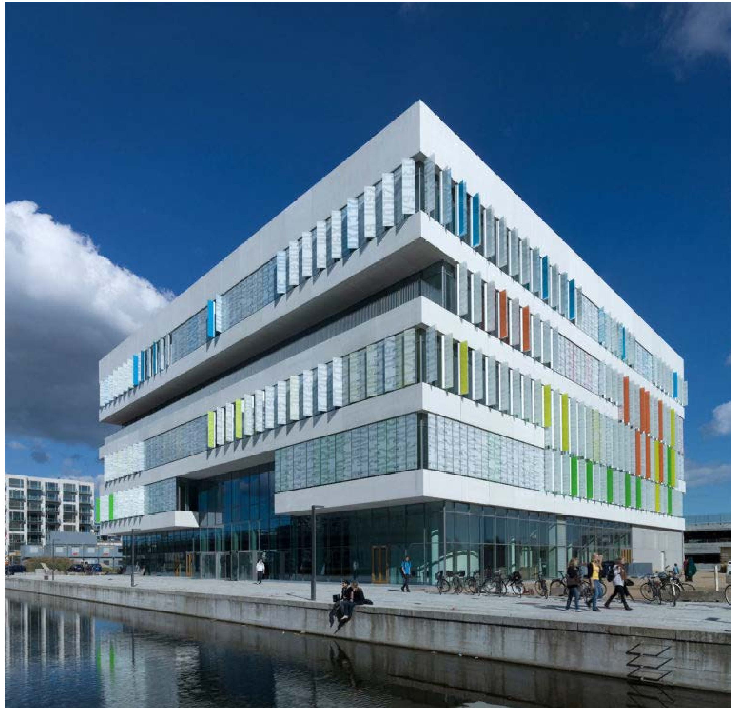
LINCOLN HIGH SCHOOL MODERNIZATION DAG 8 | MARCH 14, 2019
